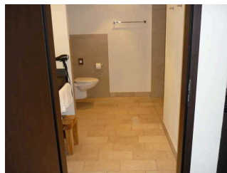
Bathroom with grab rail at the toilet
