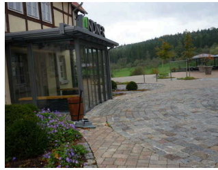
Entrance area with automatic door
