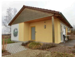
Entrance door with key code - House 5 Wood Anemone (identical in construction to House 1 Wild Garlic)
